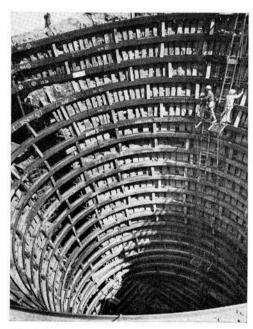
FLOOD WATER INTAKE under construction at Del Valle Dam near Livermore will release water from the reservoir during periods of high runoff in Arroyo del Valle. Water falling into this "glory hole" will drop 140 feet before turning 90° and traveling 2200 feet to the other side of the dam.
